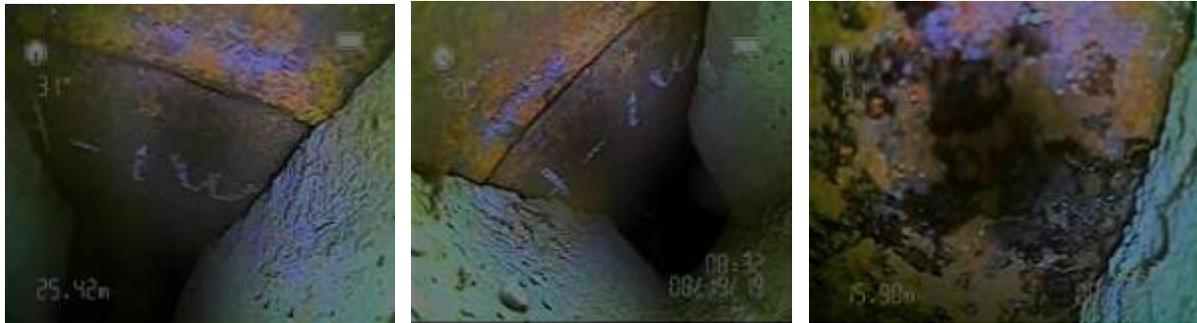
**Figure 35. Primary liner weld seams (left and center) and flakey corrosion spot (right).**
