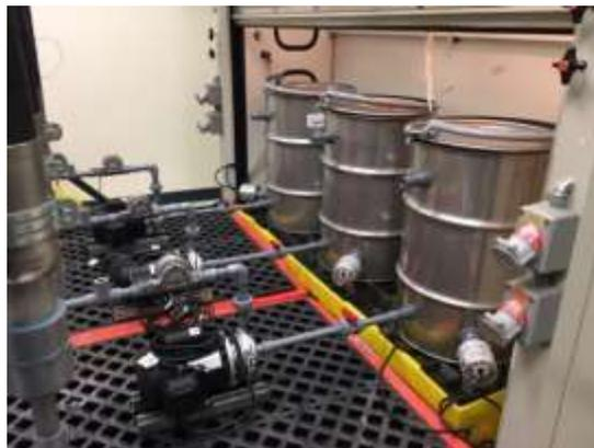
**Figure 105. Three of the system's four pumps and tanks with heaters installed.**
