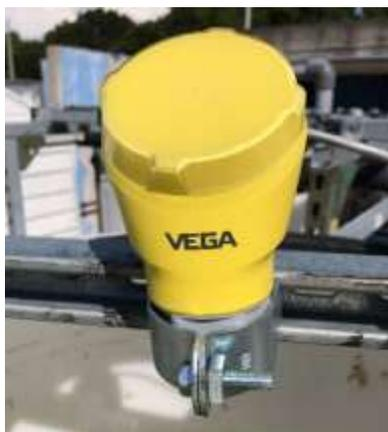
**Figure 3. Water level measurement sensor attached to the tank.**
